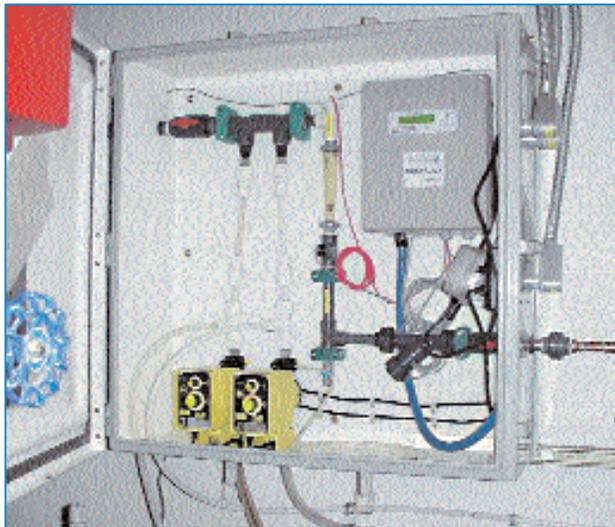
**Figure 1. A modern pre-packaged treatment pump and controller system is shown.**
